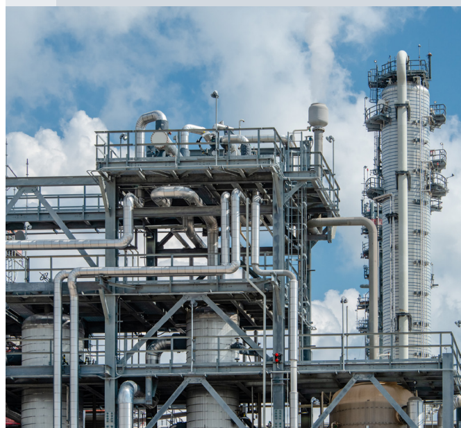
Ethane Cracker June 2019
